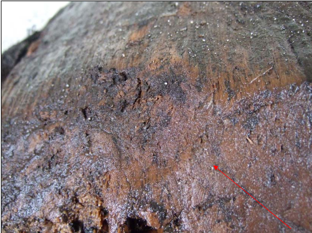
Plate 3: Timber no. 10, C17, evidence of degraded tooling.
