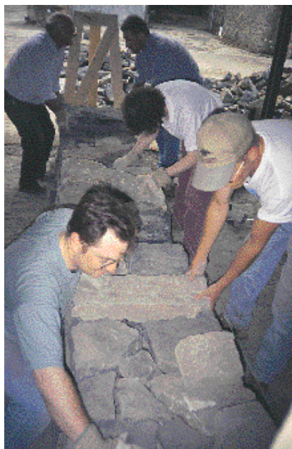
Laying through stone in double dry stone wall
