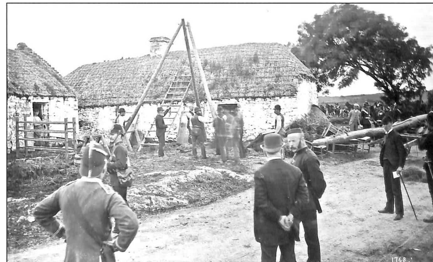
Erecting the ram at Tom Considine's eviction. Number 3 pole is positioned while Sergeant Maddox holds the swing chain. Two wooden supports seen on the left will soon be placed under the tripod. Lawrence Collection, courtesy National Library of Ireland.
